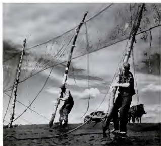
SETTING POLES in place, men then get on opposite sides of net, pull back and forth on long supporting ropes, sinking the poles to a depth of six feet.
